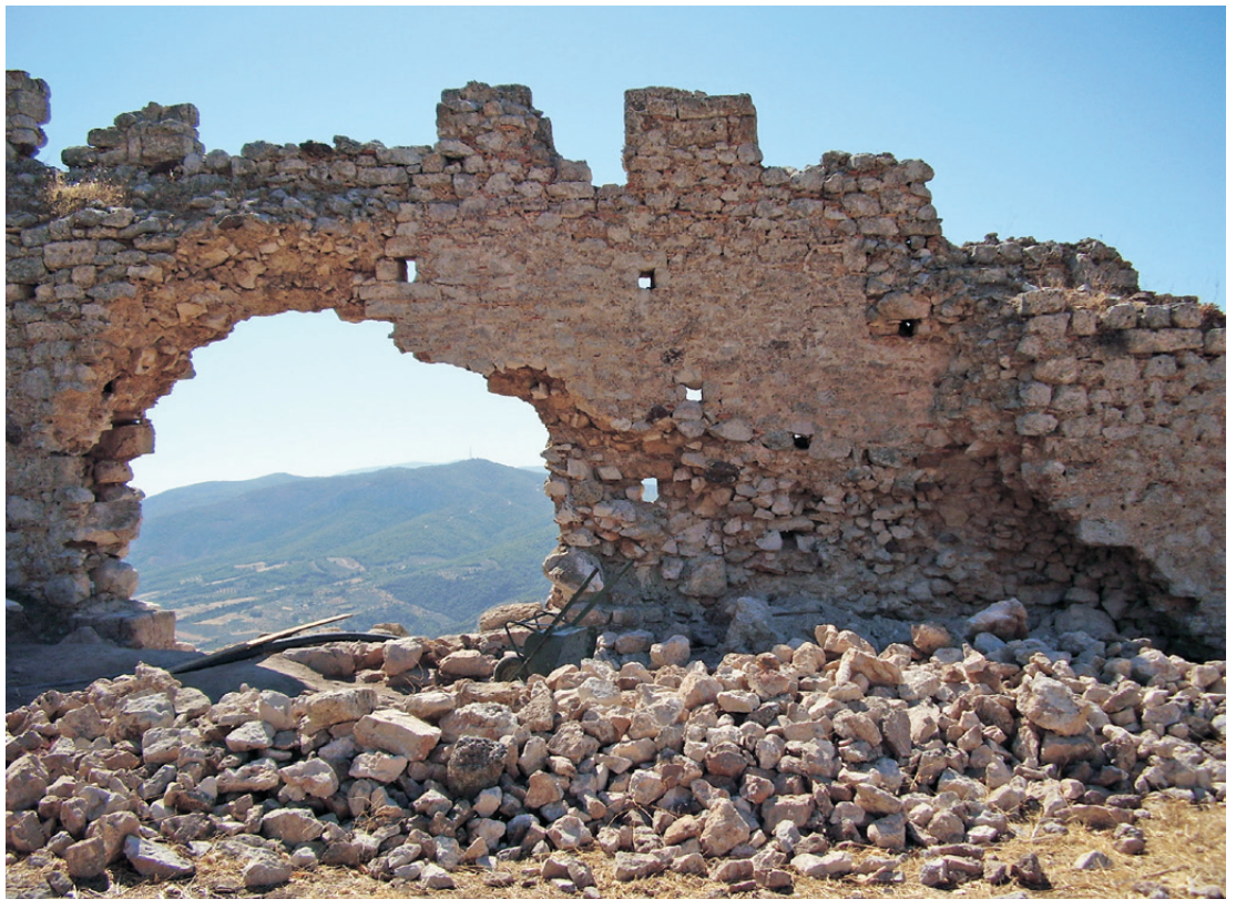
Figure 84: gate G7 before the consolidation works
