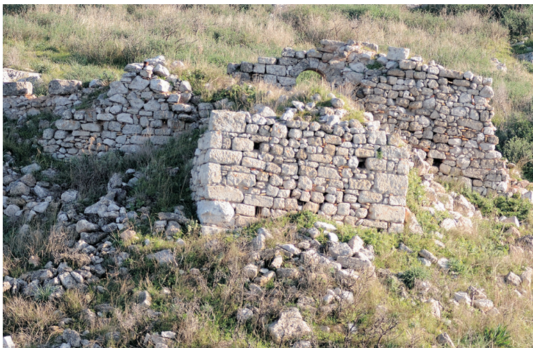
Figure 37: rectangular tower IV7
