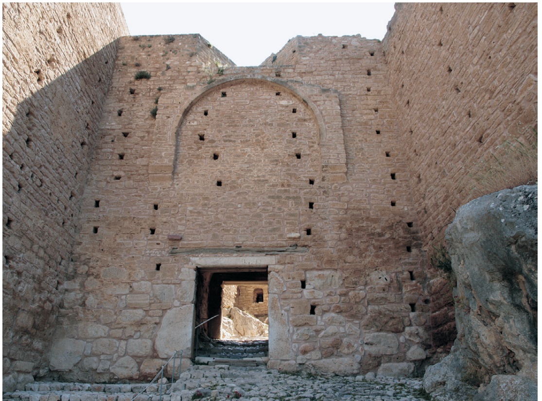
Figure 50 gate G3. Façade
