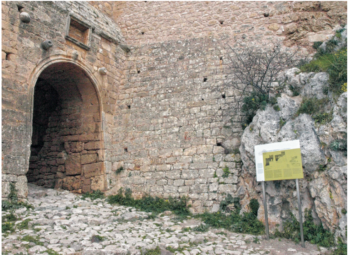
Figure 86: Gate G2 and informative sign
