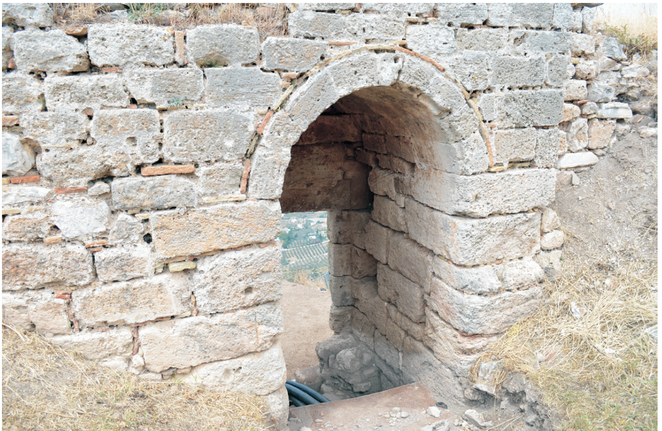
Figure 20: postern G4, from the inside
